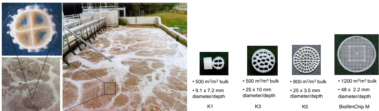
Figure 2: The moving bed biofilm reactor and various carriers supplied by AnoxKaldnes
